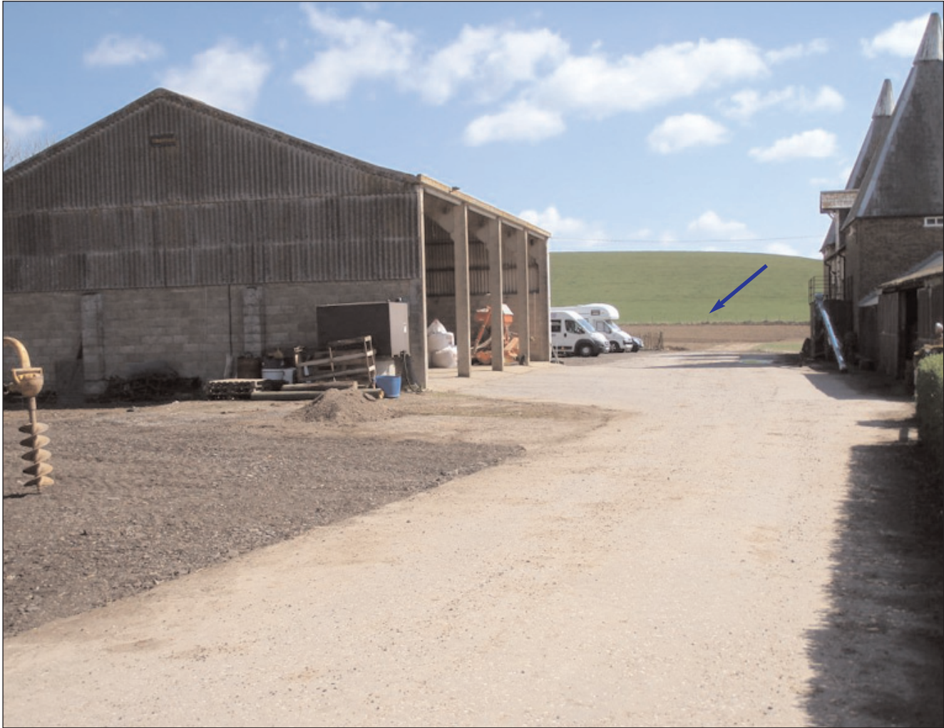
Plate 1. Looking east from the farmyard towards the proposed development site (blue arrow).
